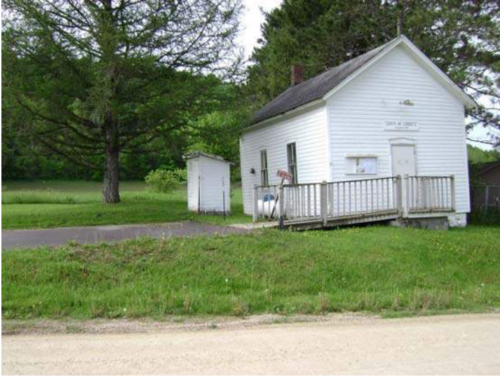
Outside photo of Town Hall after addition of handicap parking area (PHOTO 6.3)
